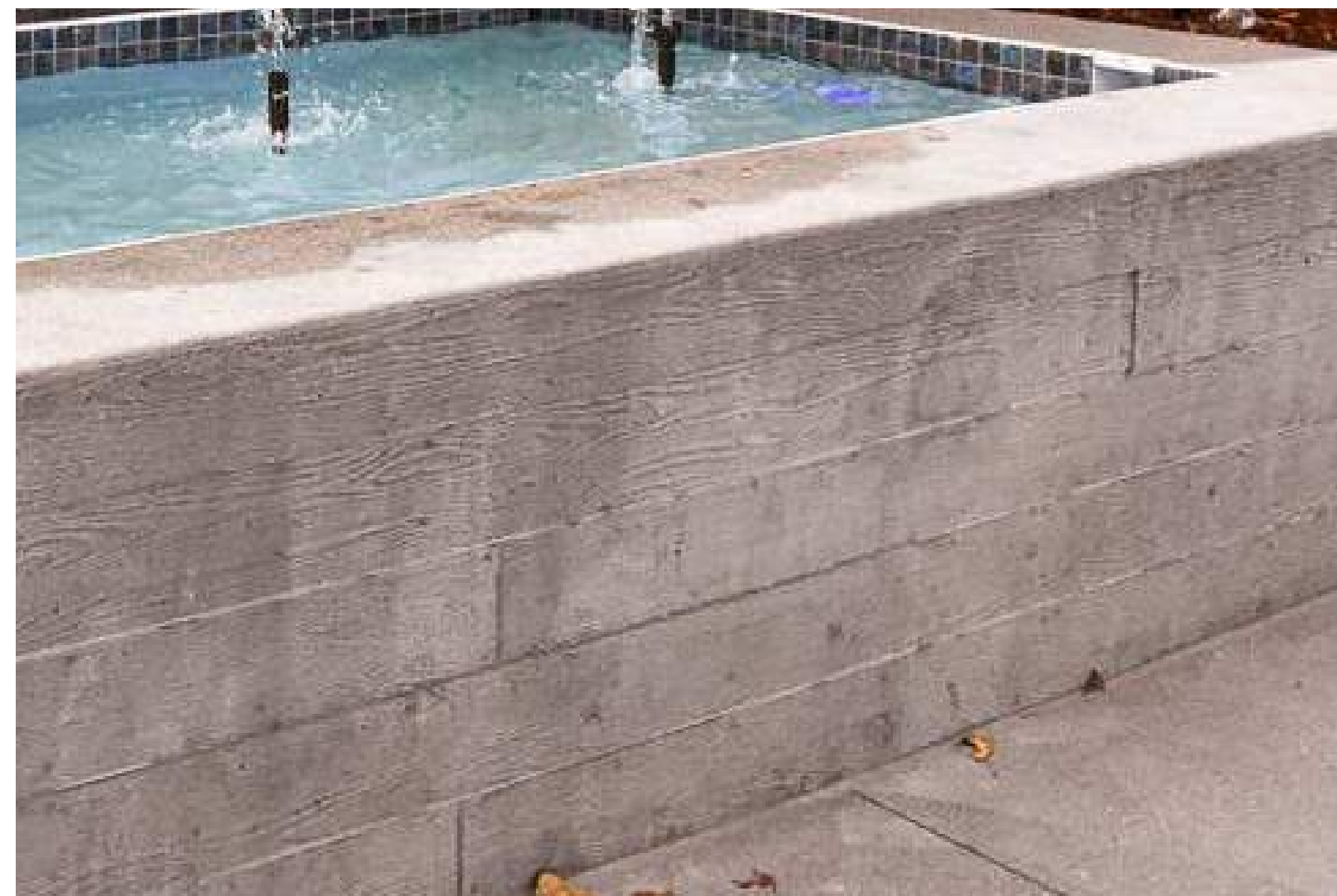
IMAGE 5 - BOARD FORMED CONCRETE
