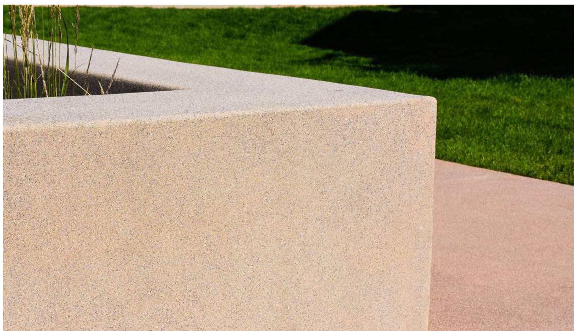
IMAGE 6 - ACID ETCH CONCRETE
