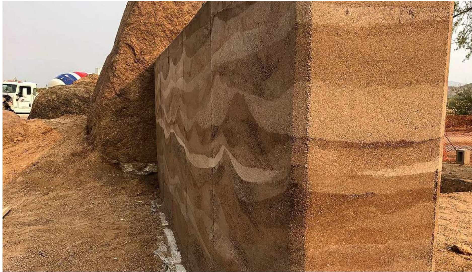
IMAGE 1 - RAMMED EARTH CONCRETE
