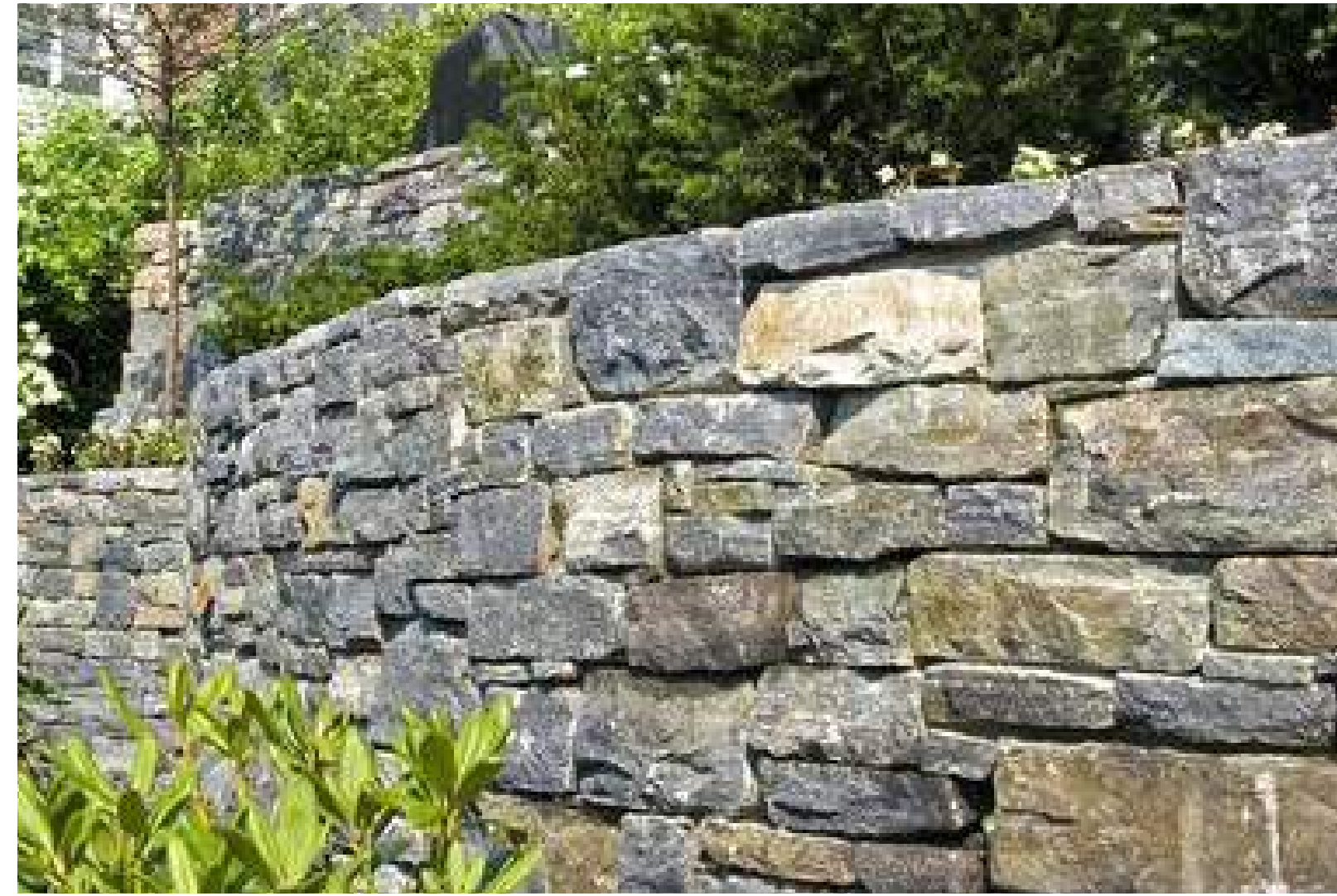
IMAGE 2 - GROUTED NATURAL STONE
